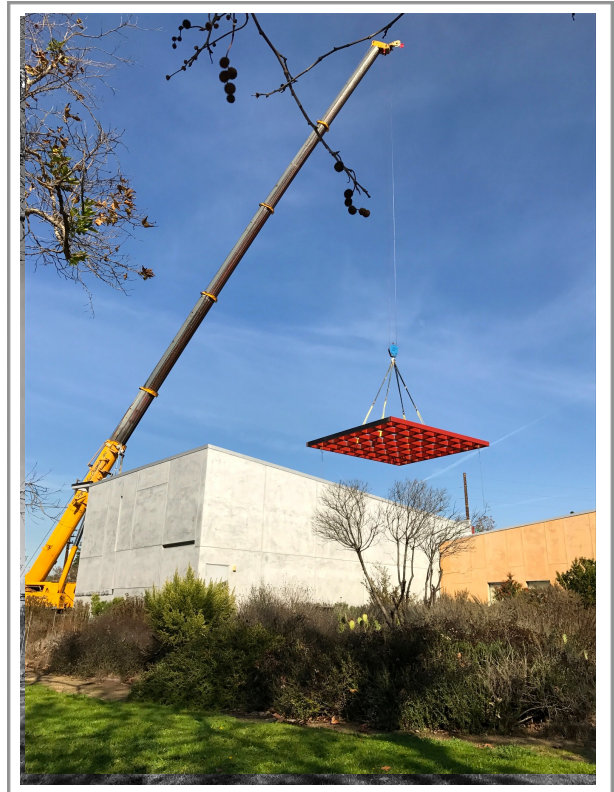
An industrial crane lifts an 18,000 pound steel lattice into position above the atrium of the Nature Center. This lattice will support glass solar panels that will provide shade as well as electricity for our center.—Photo by Bill Arrowsmith
