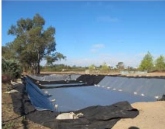
*Construction of new subsurface biofilter begins with a 110'x35'x6' hole, lined with fabric to form water barrier.*
