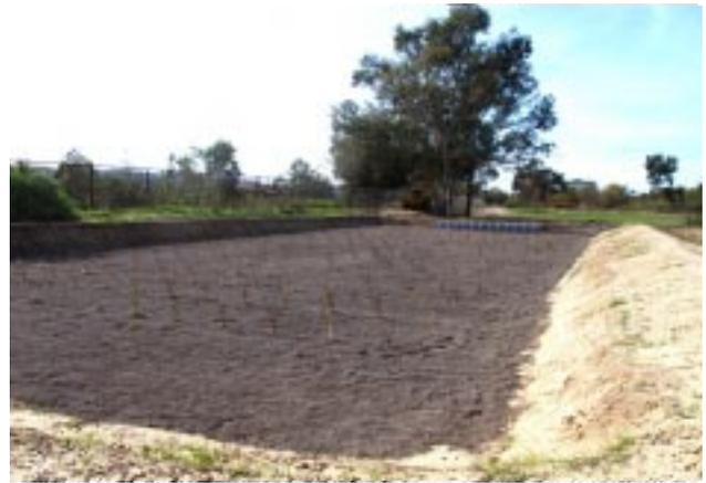
*Biofilter complete with special Vetiver grass from India planted. Twelve pipes protruding at far end supply water that has been pumped up from the sump.*
