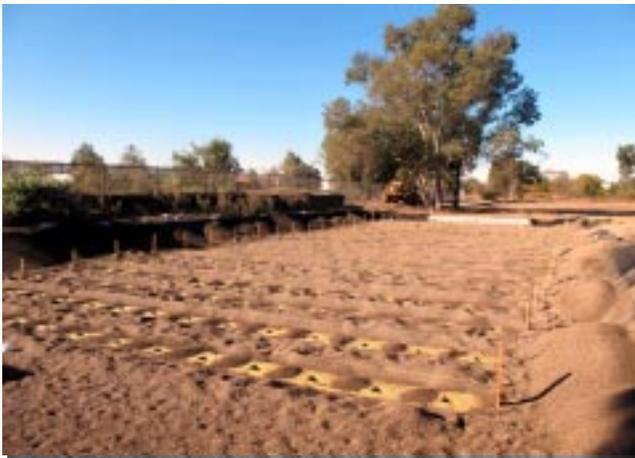
*The hole is then filled with adsorbent gravel-like stone plus rows of special absorbent media (lighter boxes) in which grass will be planted.*
